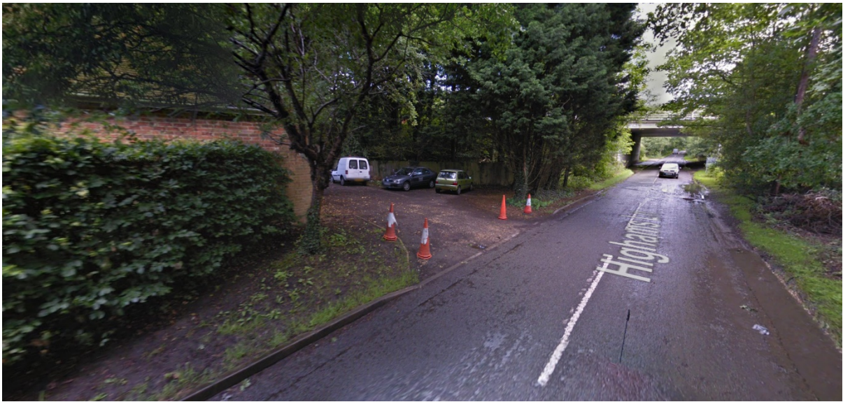
Existing Bridleway Access
